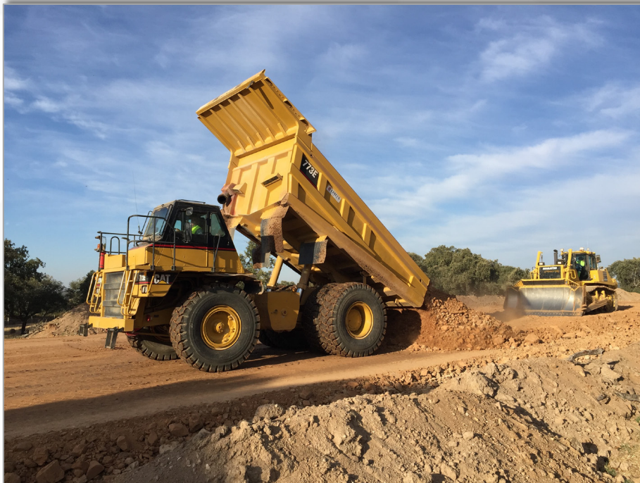
Mine contractors constructing the new 5 kilometre road at the Salamanca project in Western Spain
